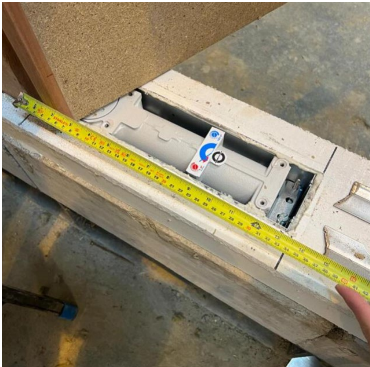
Photo C.3 – Closer (floor spring), showing cover removed during installation for surveying purposes..
